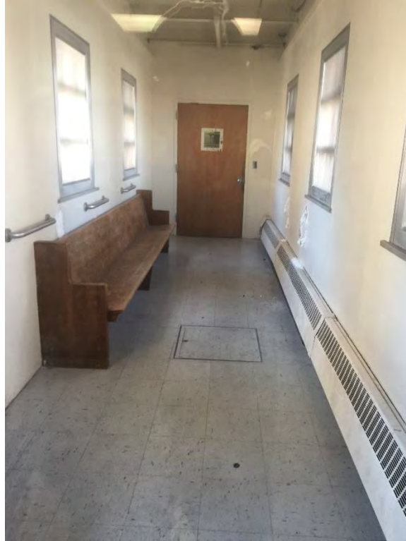
Bridge Interior – No Access
