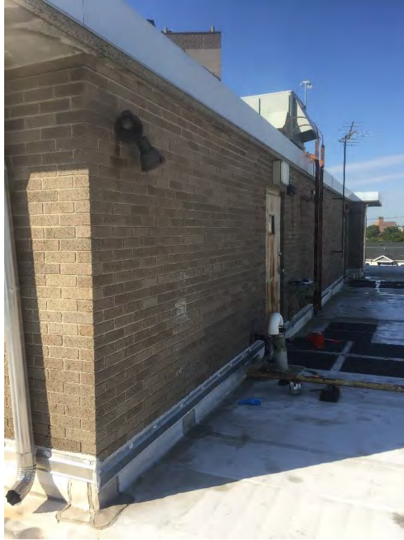
Upper Roof A Access
