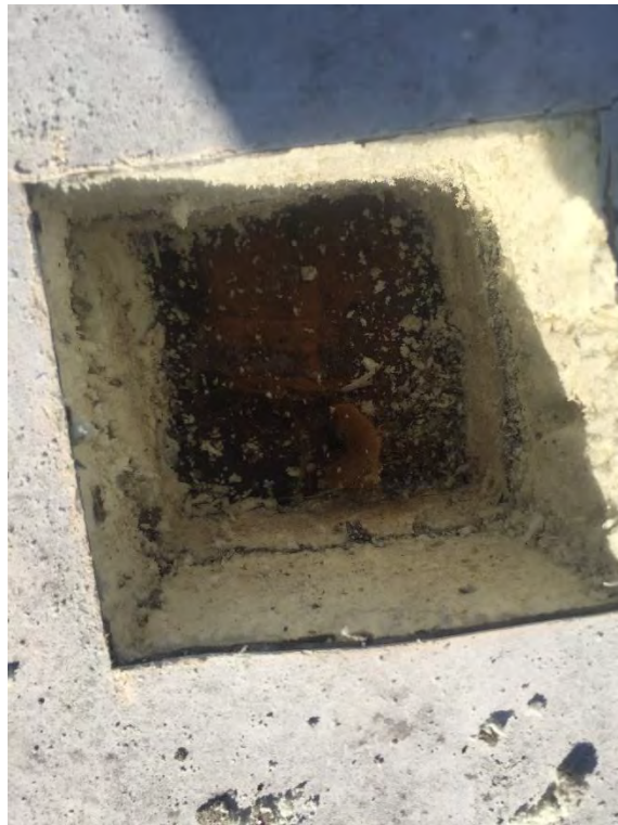
Upper Roof A Sample
