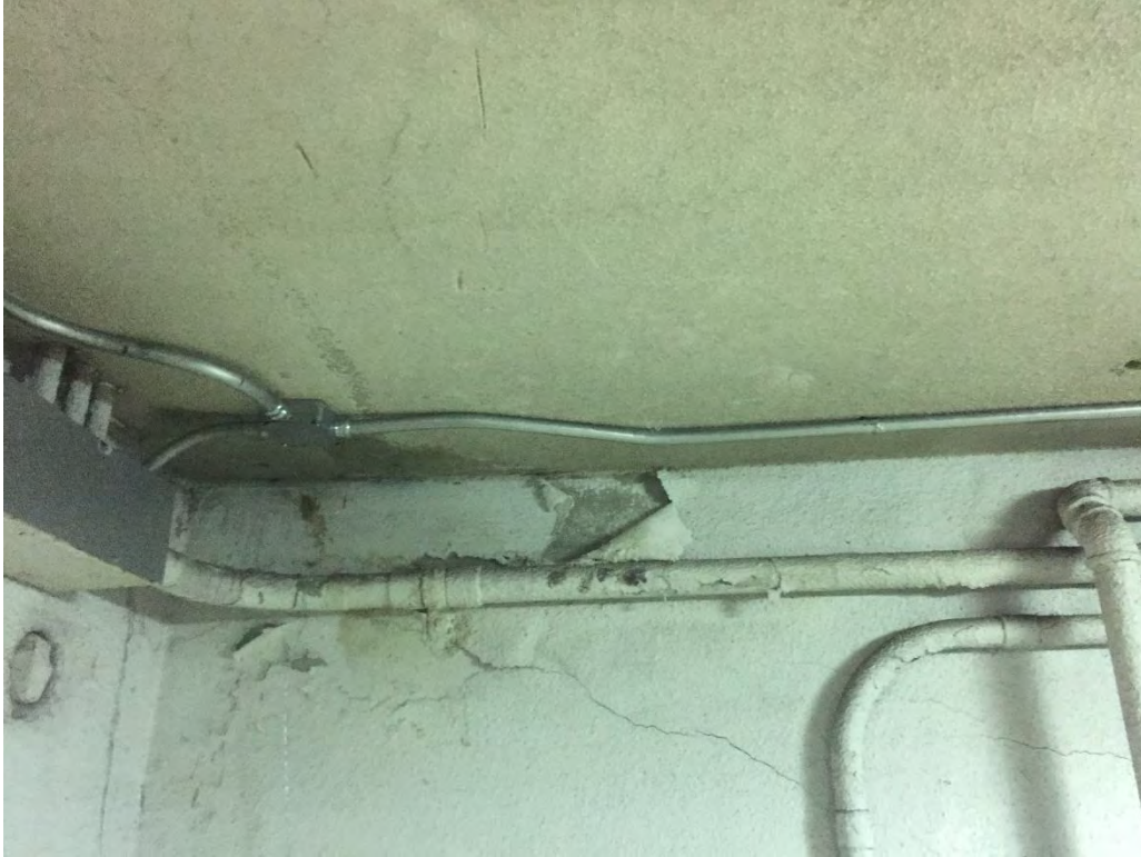
Wall Stucco Ceiling
