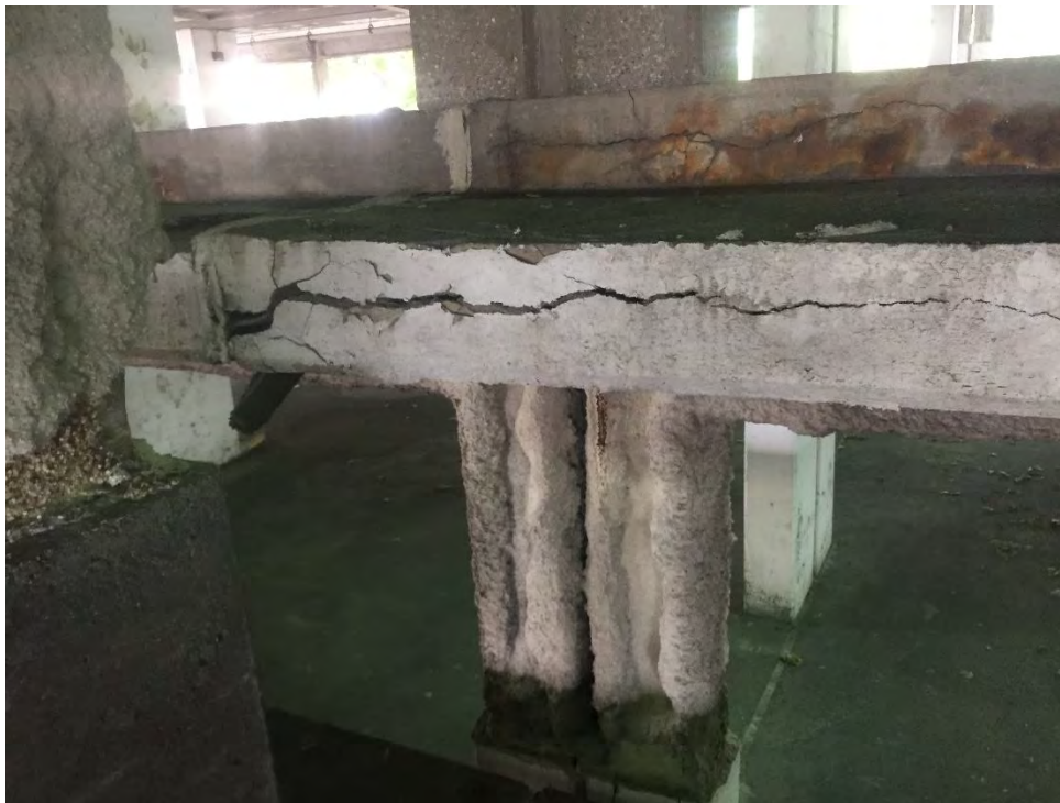
Concrete Decking SOFP
