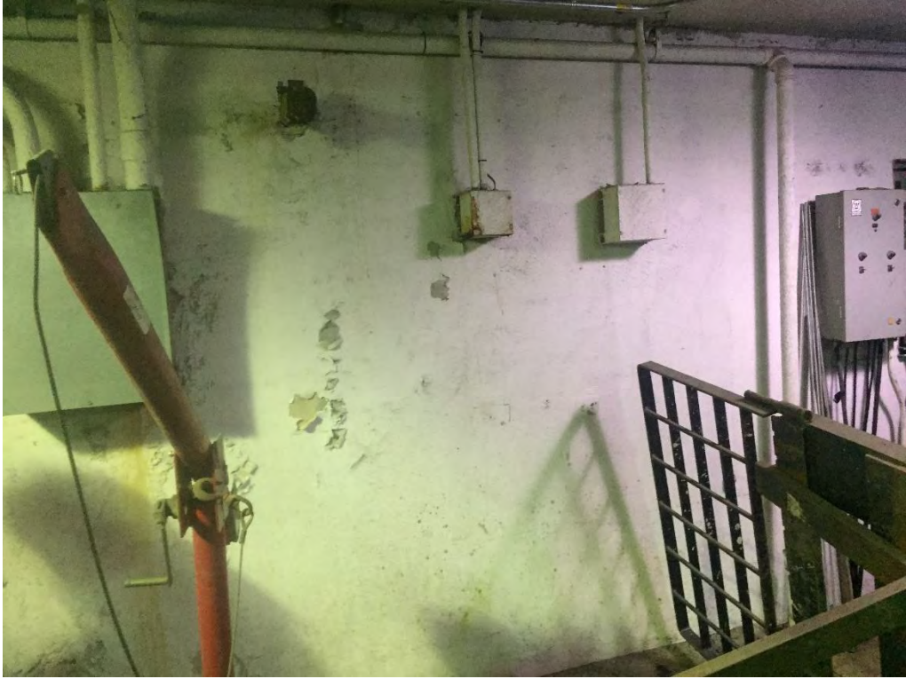
Wall Texture Stucco
