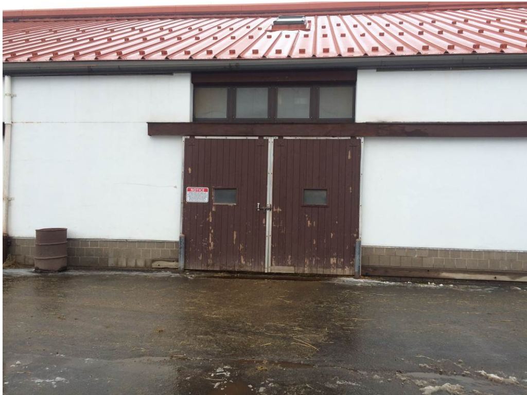
Photograph 1: Existing Barn Style Door with Window
