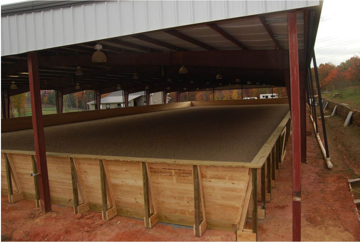
Sample Construction Photo 4
