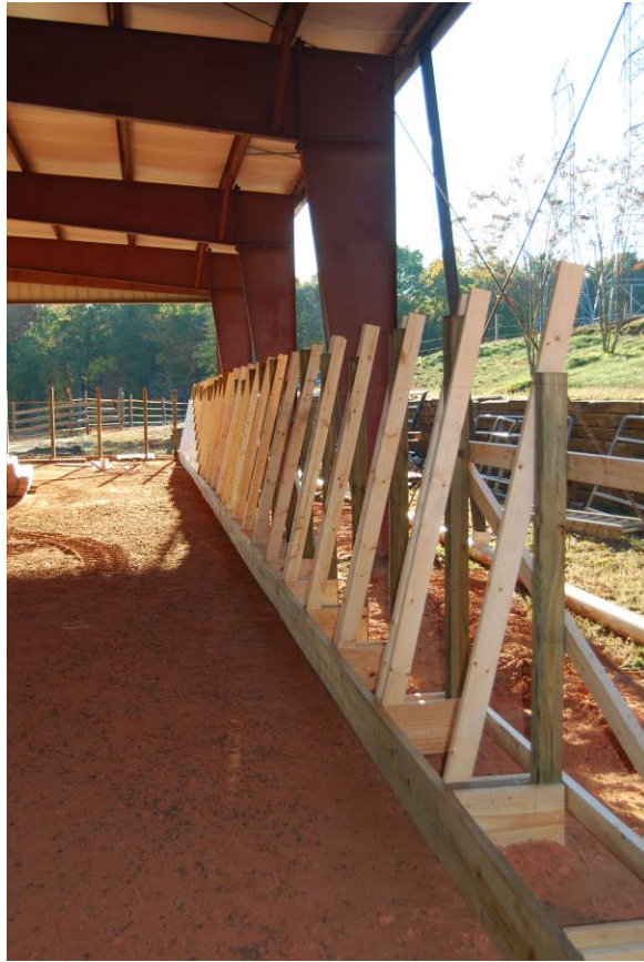
Sample Construction Photo 2
