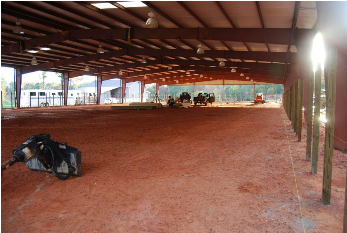
Sample Construction Photo 1
