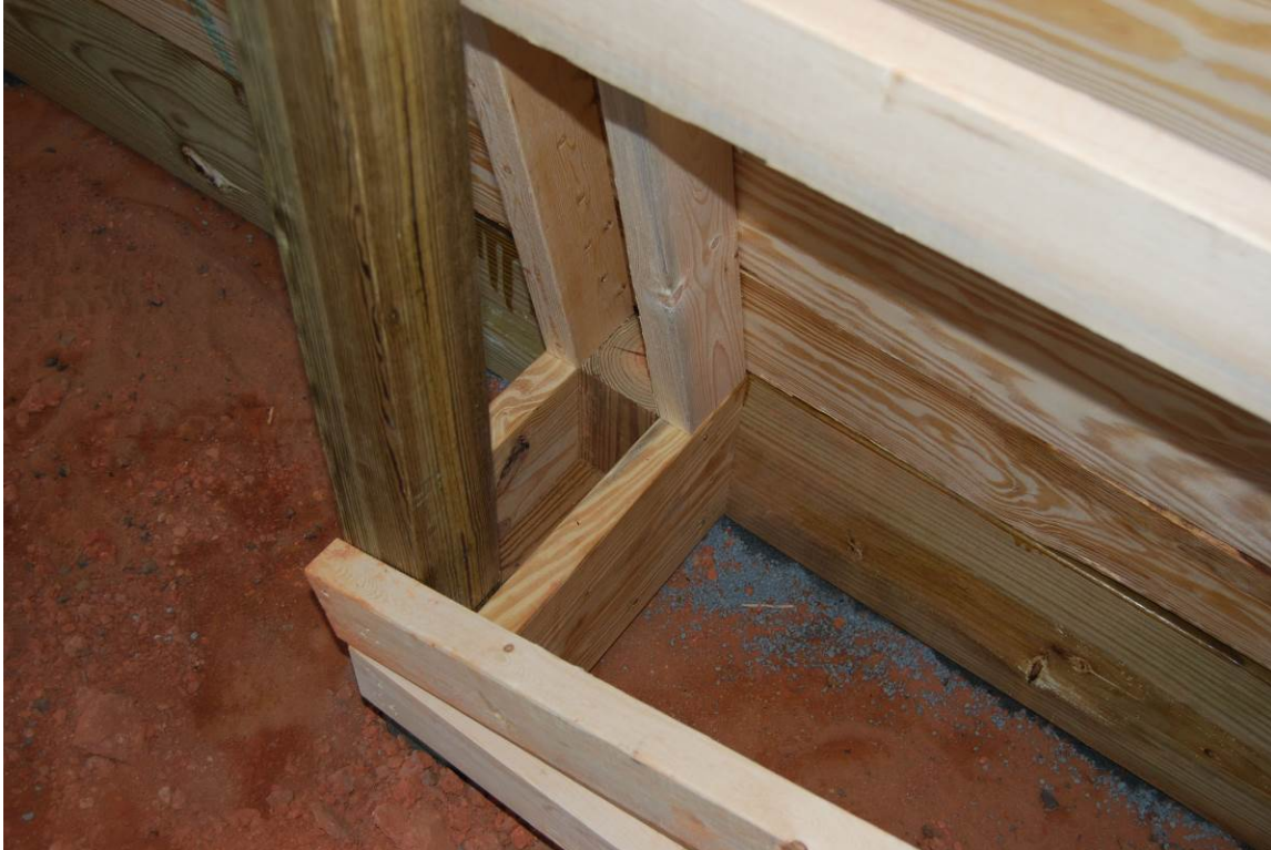
Sample Construction Photo 3
