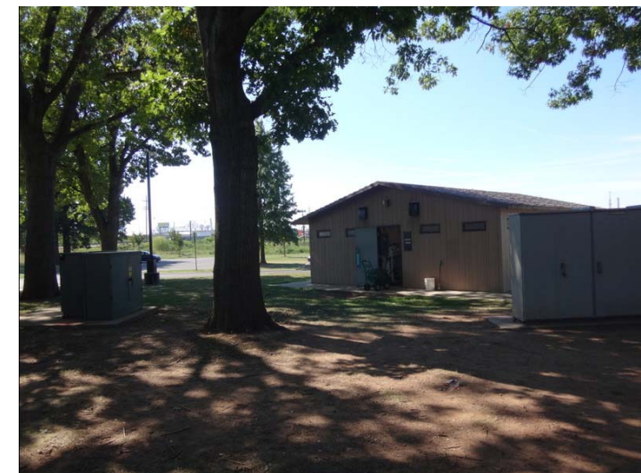
PHOTO B - FIELD HOUSE UTILITY ROOM Existing Field House Building
