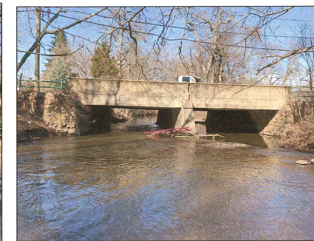
LOCATION 22: SOUTH BRIDGE ELEVATION, LOOKING NORTH
