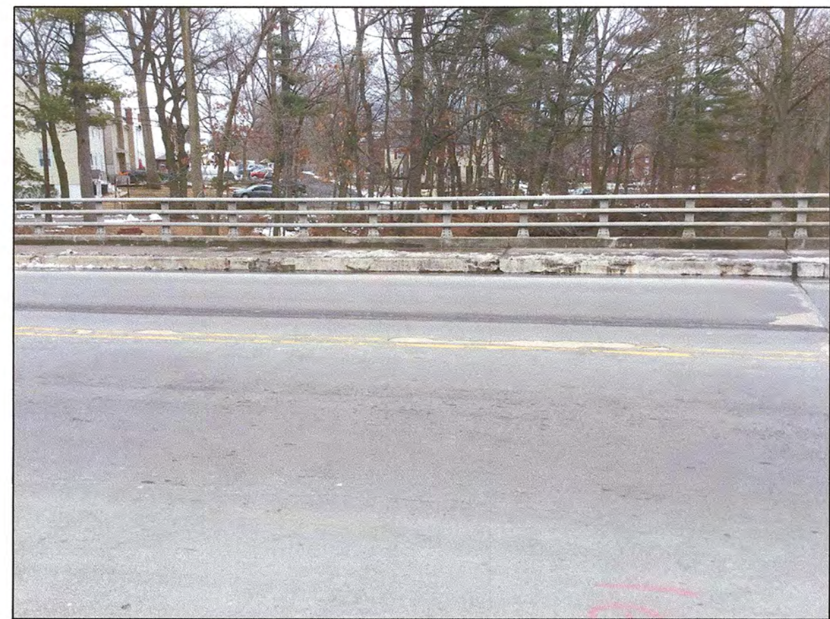
LOCATION 20: BRIDGE DECK, LOOKING NORTH
