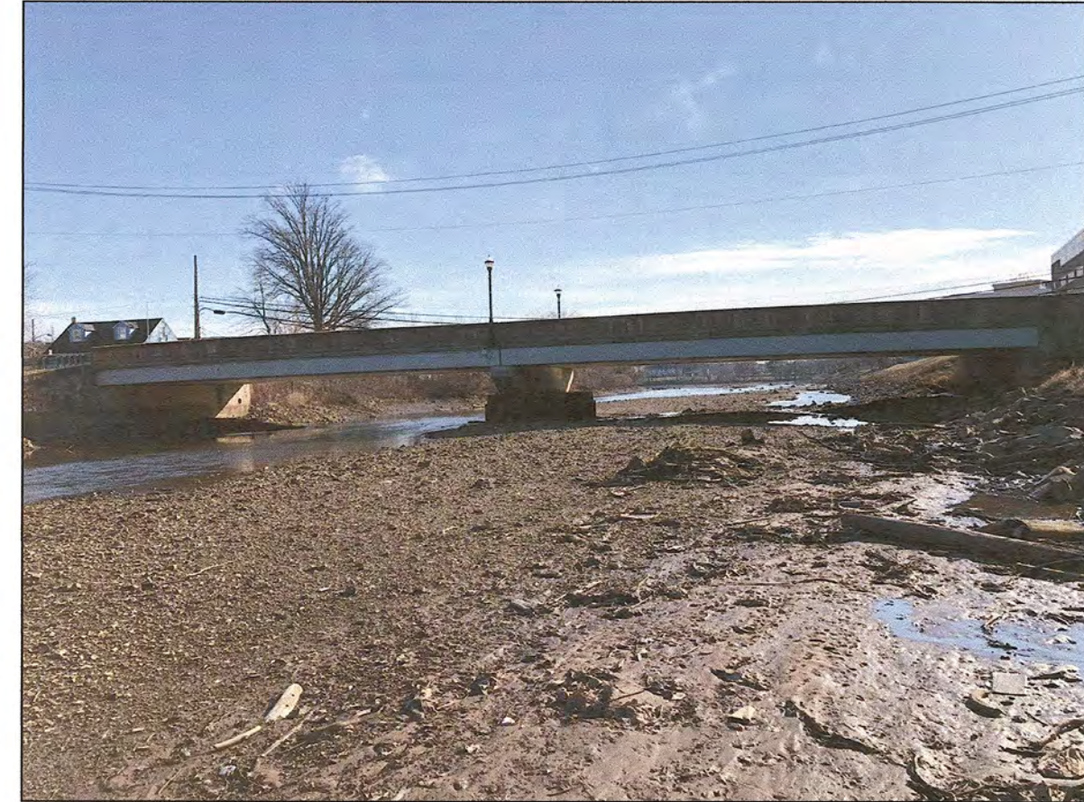
PICTURE LOCATION: SOUTH BRIDGE ELEVATION, LOOKING NORTH
