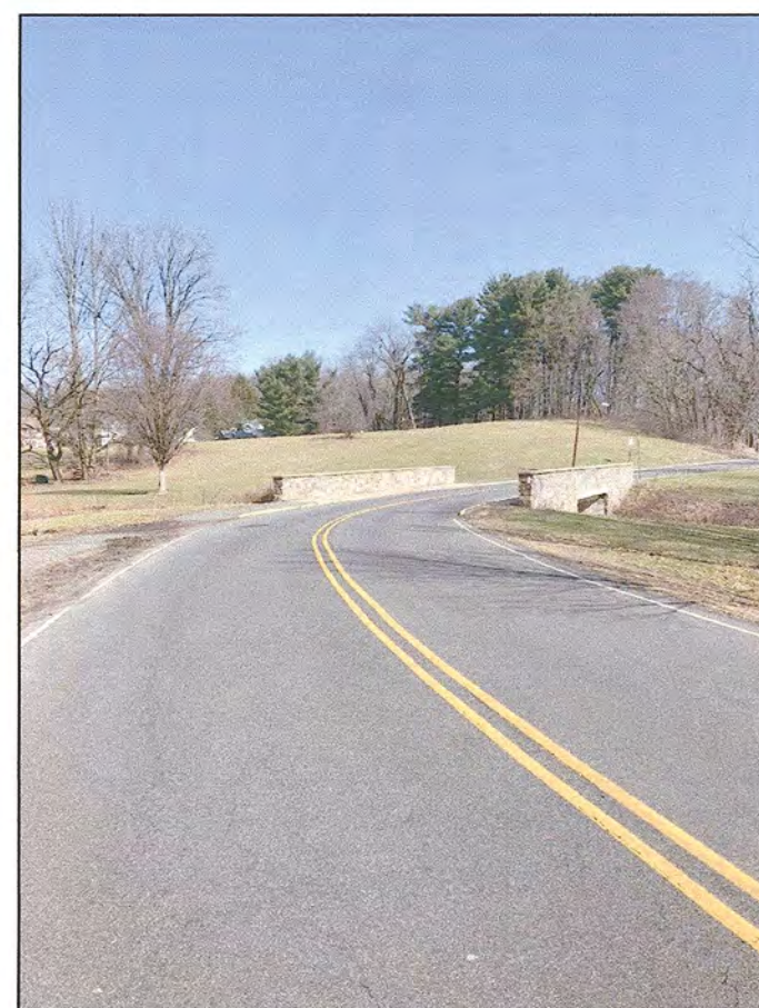
PICTURE LOCATION: WEST BRIDGE APPROACH LOOKING EAST
