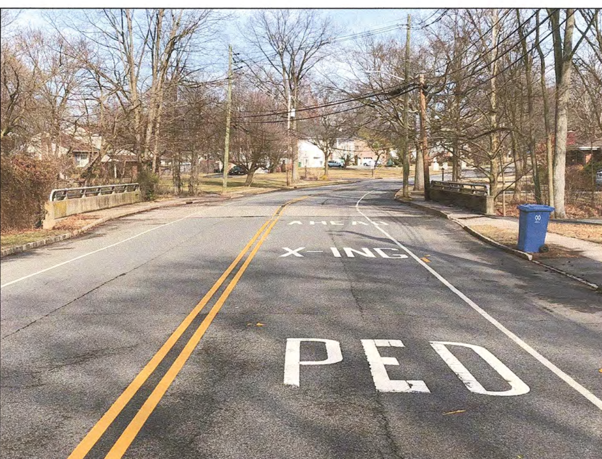
PICTURE LOCATION: TAKEN UPSTREAM FACING DOWNSTREAM WHERE DEBRIS BUILDS UP AT UTILITY PIPE CROSSING.
