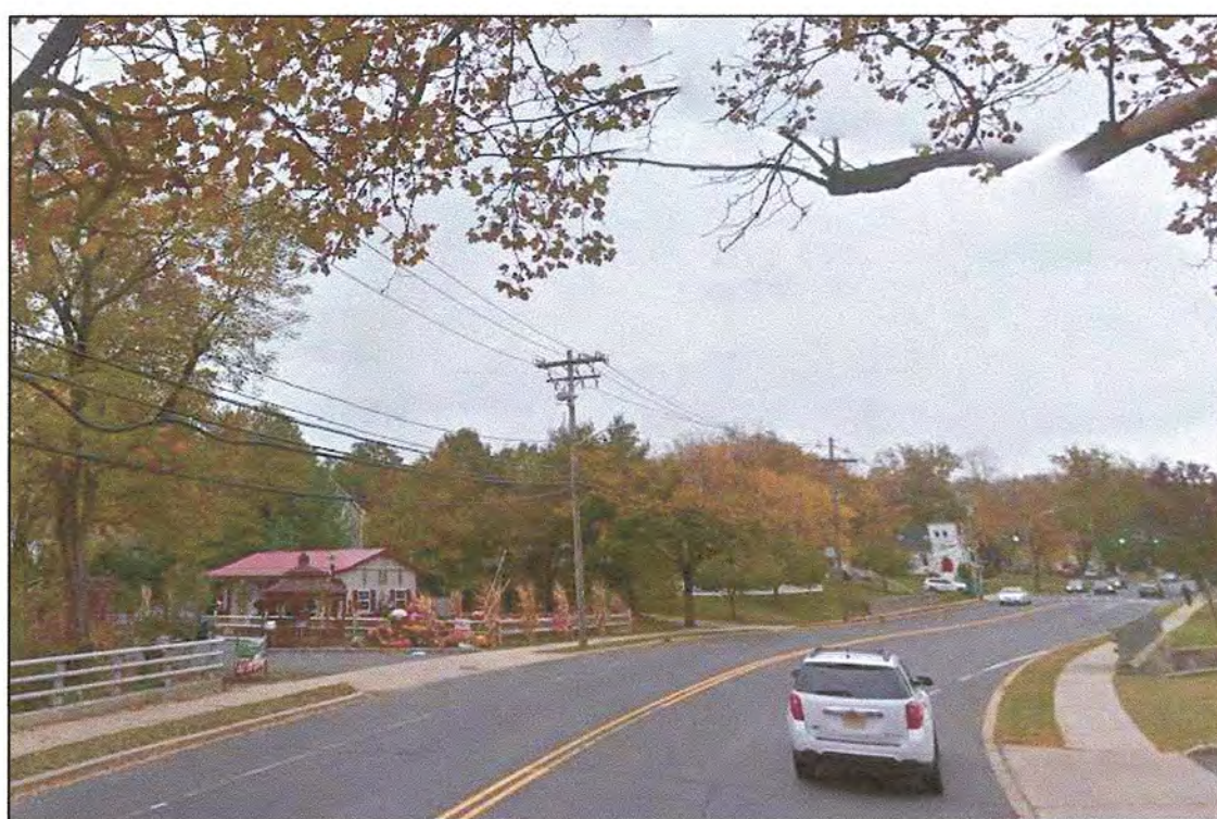
PICTURE LOCATION: TAKEN FROM THE NORTH BRIDGE ABUTMENT, LOOKING SOUTH
