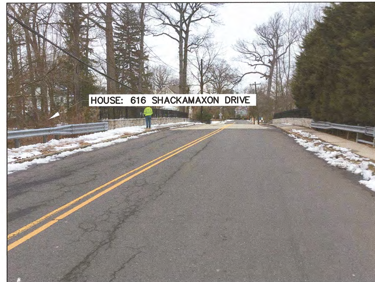
LOCATION 21: EAST BRIDGE APPROACH, LOOKING WEST
