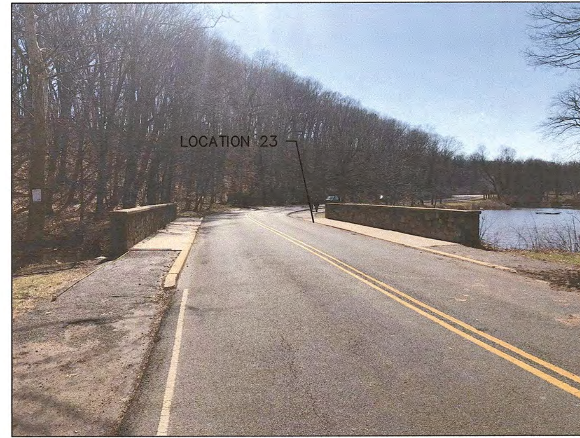
PICTURE LOCATION: PICTURE TAKEN ALONG PARK DRIVE FACING SOUTHWEST.
