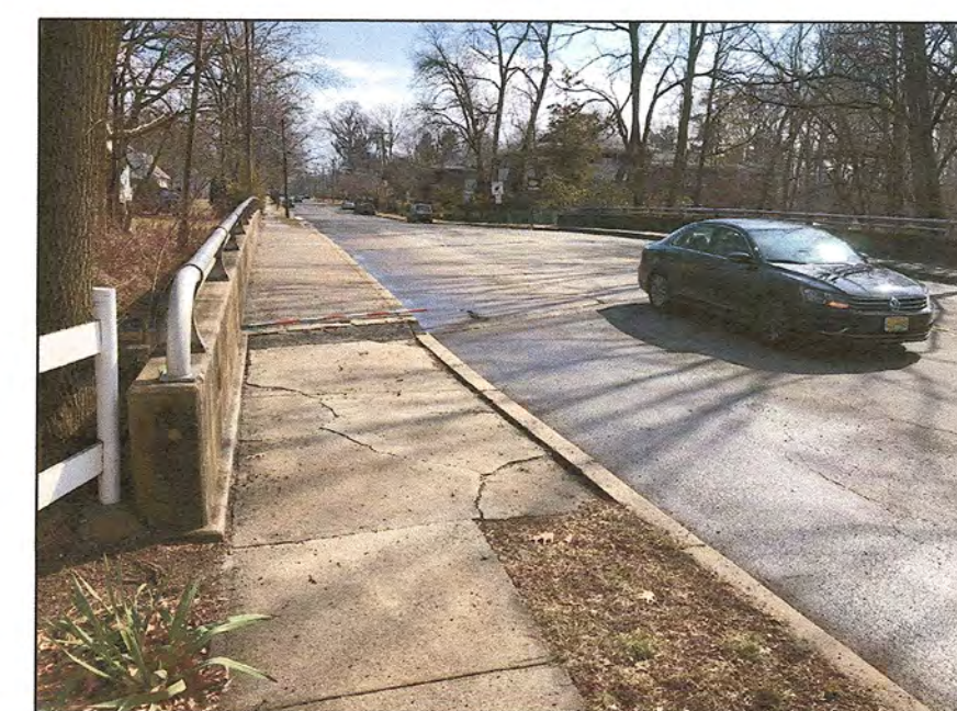
NORTHWEST APPROACH SIDEWALK, LOOKING EAST.
