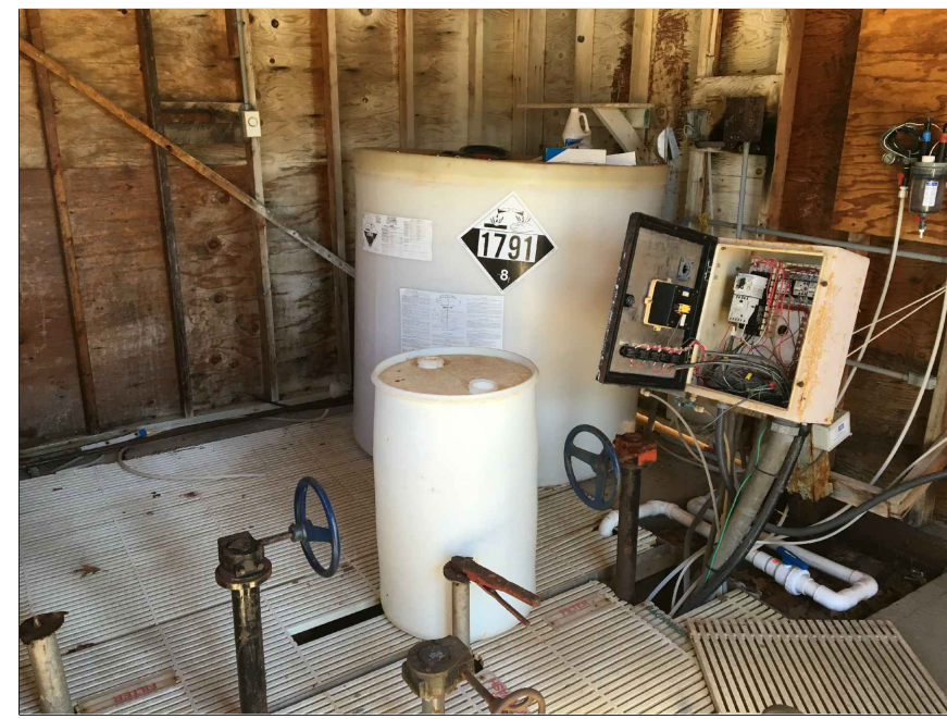
5. INTERIOR OF FILTER BLDG.
