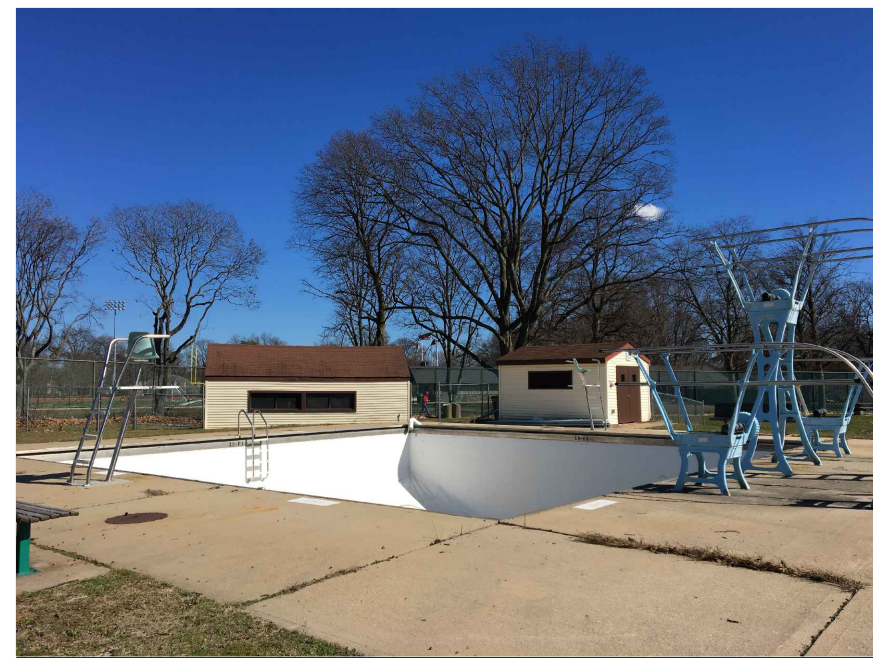
1. OVERVIEW OF DIVE TANK AREA
