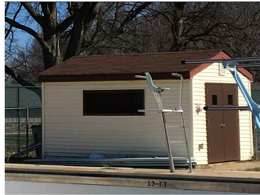
3. EXTERIOR OF FILTER BLDG.
