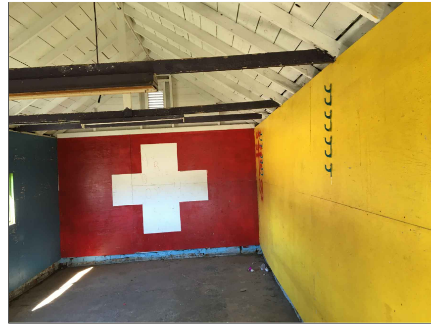
7. INTERIOR OF LIFE GUARD BLDG.
