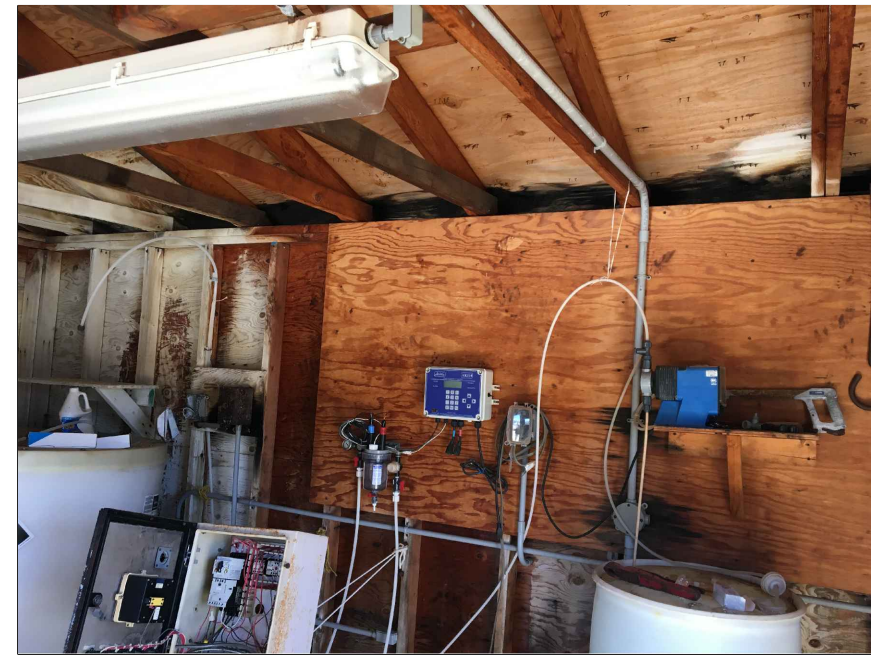
6. INTERIOR OF FILTER BLDG.
