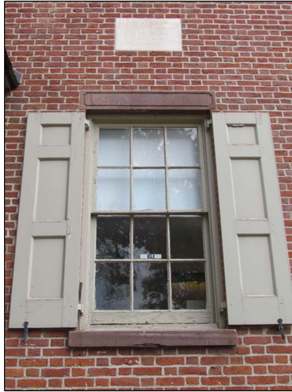
Figure 17: Typical conditions seen on window 110.
