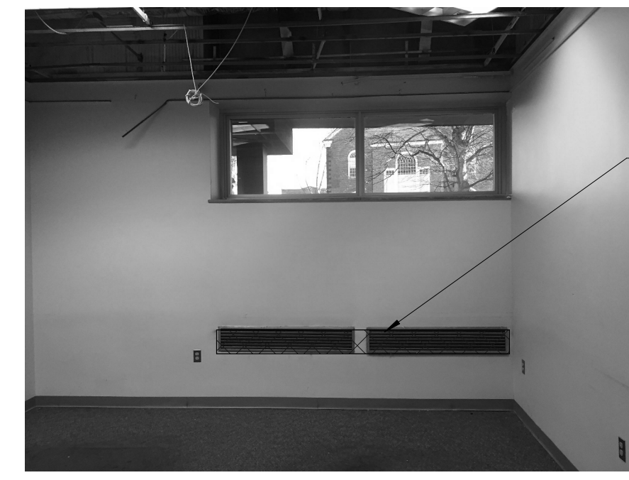
3 PHOTO 1 - DEMOLITION (BY GC)
