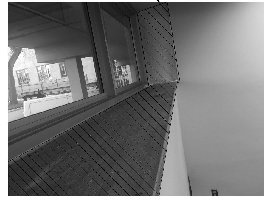
5 PHOTO 3 - NEW WORK (BY OWNER)
