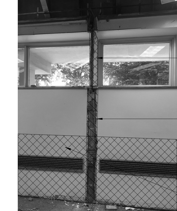
6 PHOTO 4 - NEW WORK (BY OWNER)
