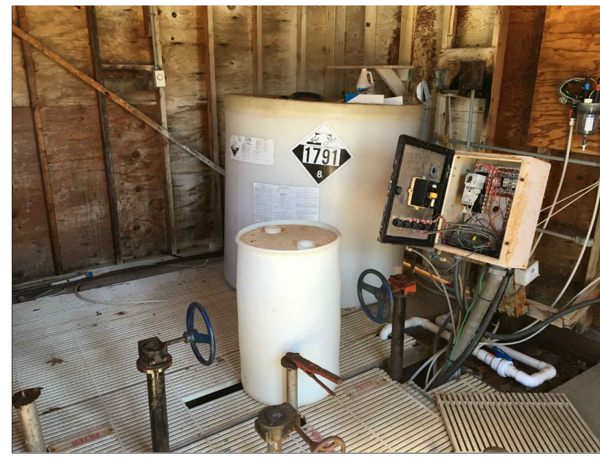
5. INTERIOR OF FILTER BLDG.
