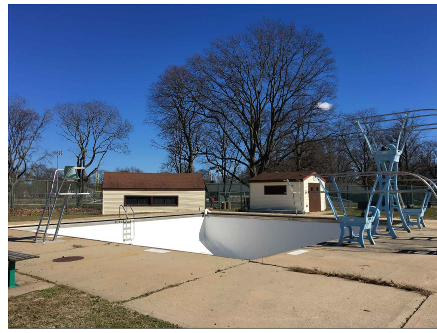
1. OVERVIEW OF DIVE TANK AREA
