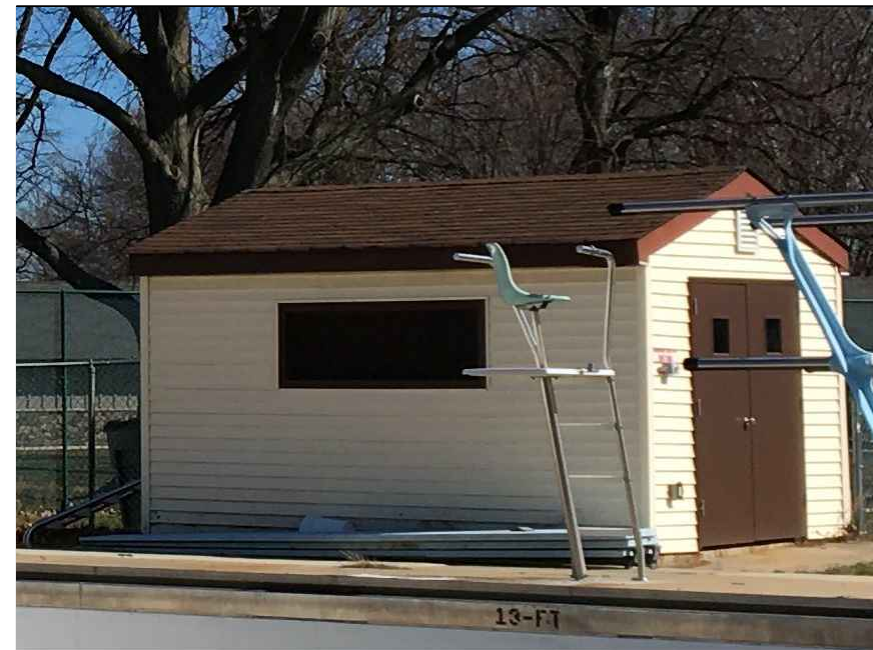
3. EXTERIOR OF FILTER BLDG.
