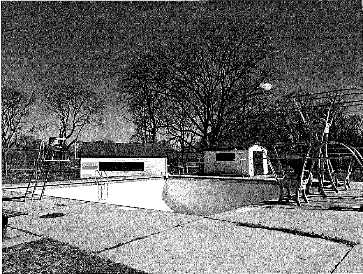
Photograph 1: Site Overview of Dive Tank (Pool) Area
