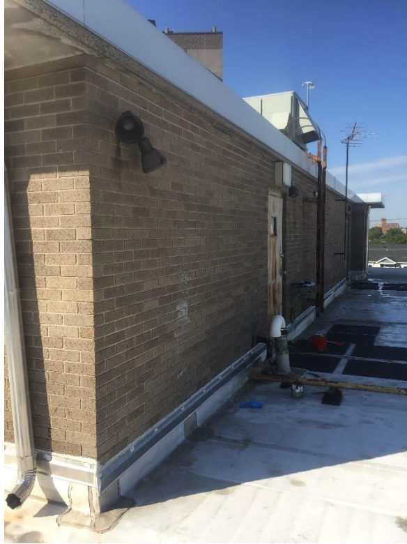
Upper Roof A Access
