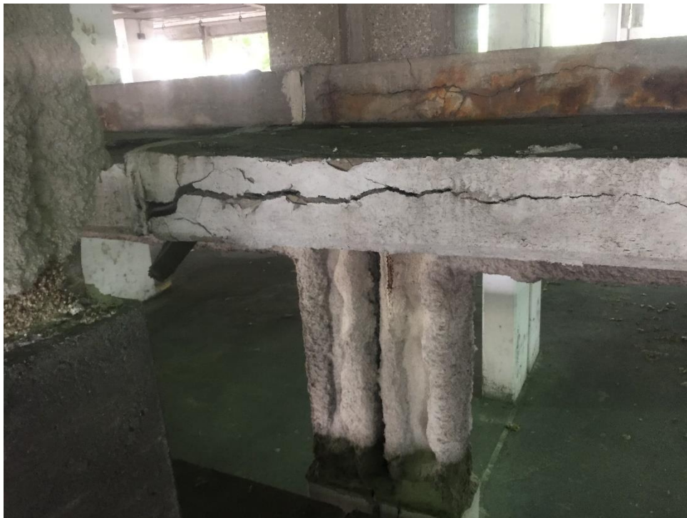
Concrete Decking SOFP
