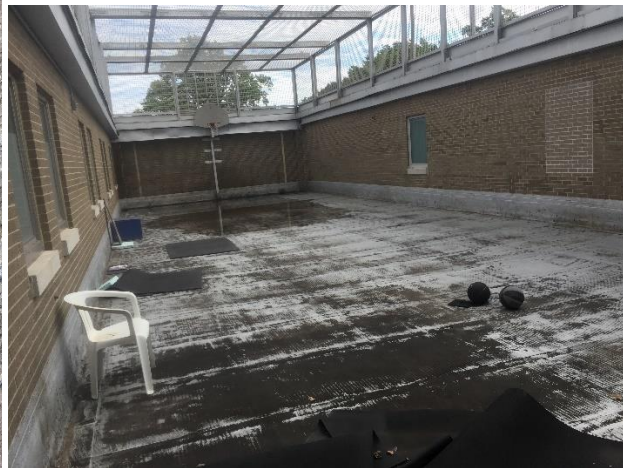
Roof top prison yard
