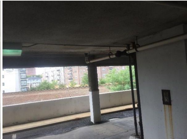
ACM Stucco ceiling
