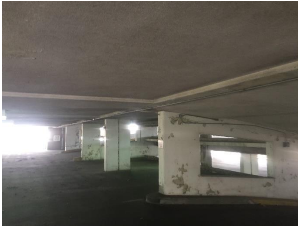
ACM Stucco ceiling
