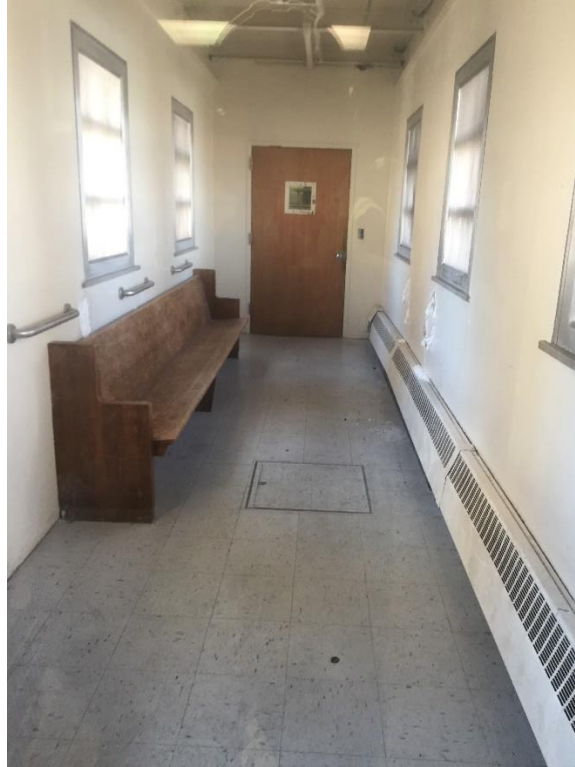
Bridge Interior – No Access
