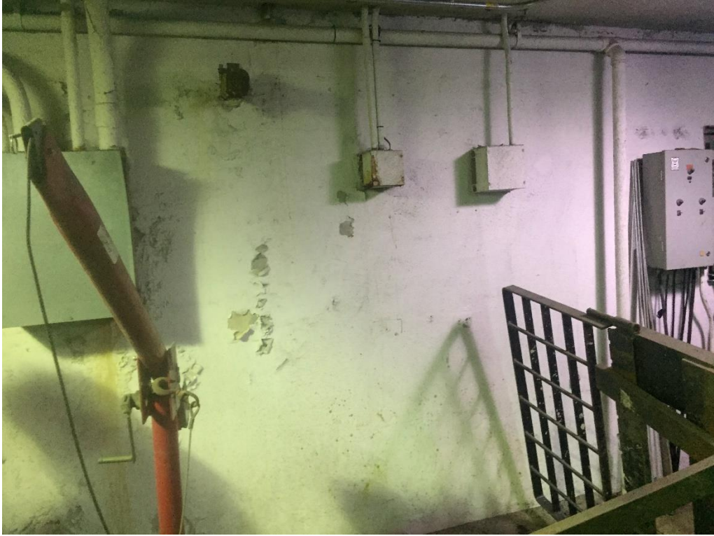
Wall Texture Stucco
