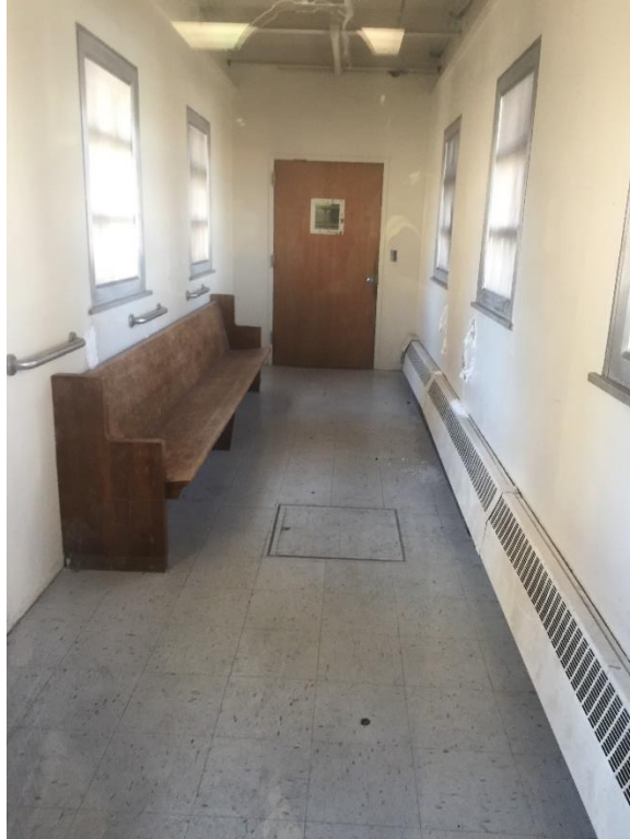
Bridge Interior – No Access
