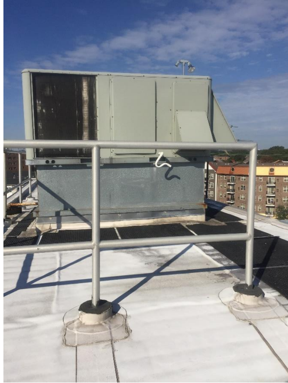
Upper Roof A
