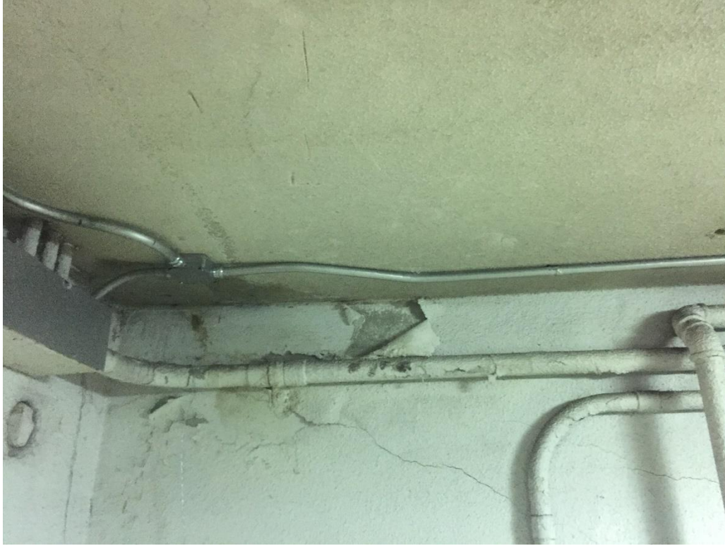
Wall Stucco Ceiling
