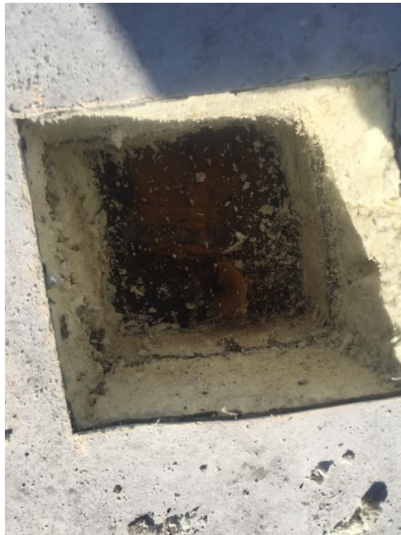
Upper Roof A Sample
