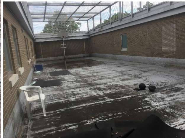
Roof top prison yard
