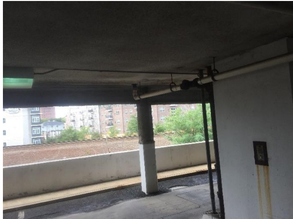
ACM Stucco ceiling
