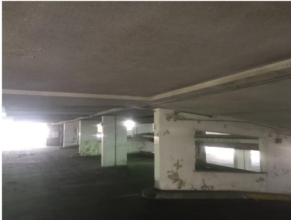
ACM Stucco ceiling
