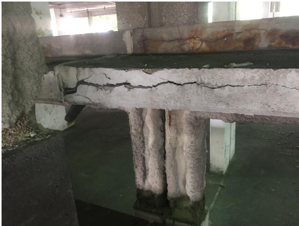
Concrete Decking SOFP
