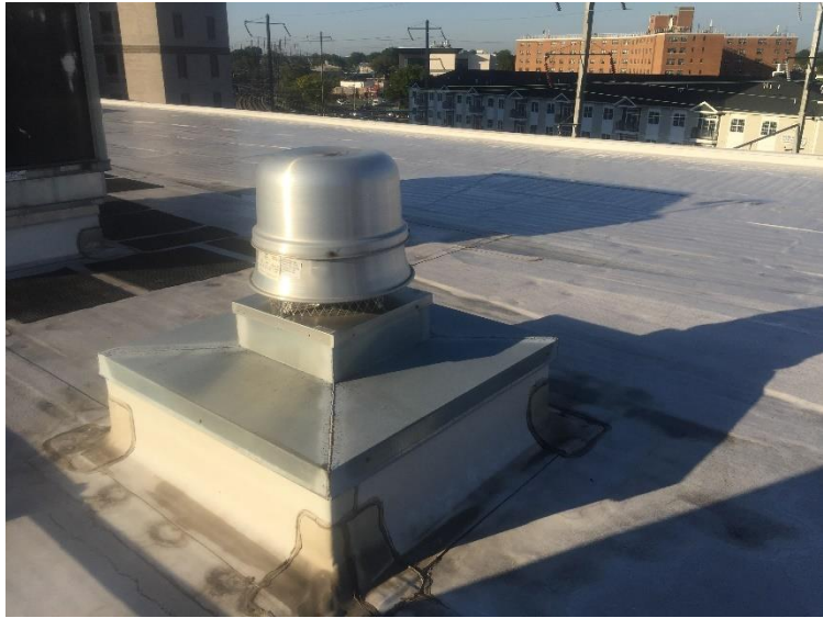
Vent flashing
