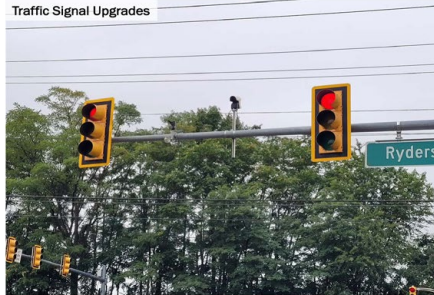
Traffic Signal Upgrades
