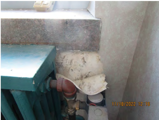
Photographs 6 & 7 – 12 th Floor Corner Office Mold on Wallpaper adjacent to Window
