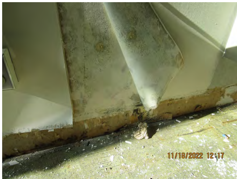
Photograph 9 – 12 th Floor Corner Office Mold on Sheetrock Behind Wallpaper on Shared Wall Between Bathroom and Office
