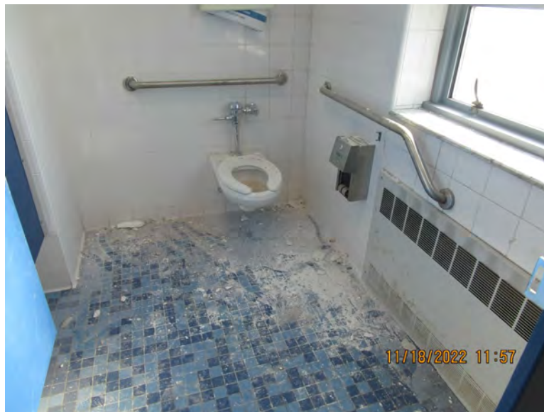
Photograph 2 – 12 th Floor Men's Restroom Plaster Debris on Floor
