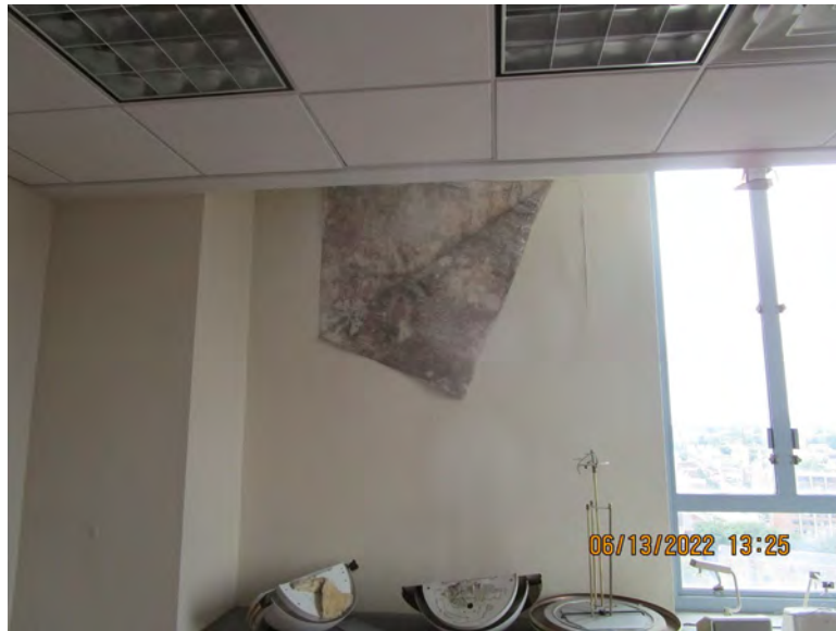
Photograph 10 – 13 th Floor Suspect Mold Growth on Sheetrock Behind Delaminating Wallpaper
