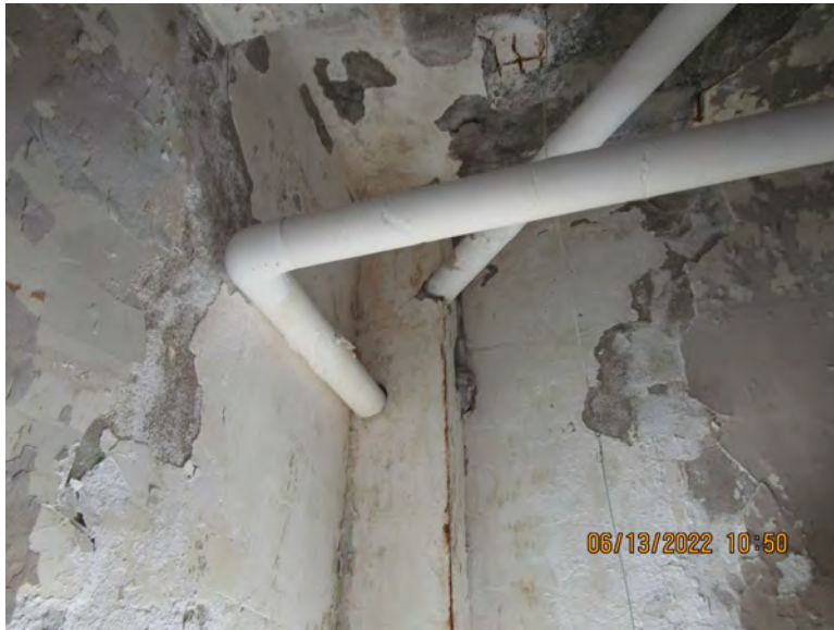
Photograph 3 – Two (2) Pipes Entering Chase on 15 th Floor Fiberglass Insulated Pipe in Foreground
