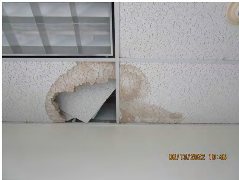
Photograph 2 – 15 th Floor Water Damaged Ceiling Tile
