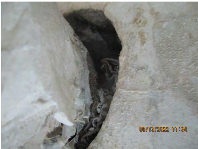
Photographs 4 – Compressed Paper Insulation (ACM) at Penetration into Chase (Assume All Compressed Paper Insulation in the Chase)
