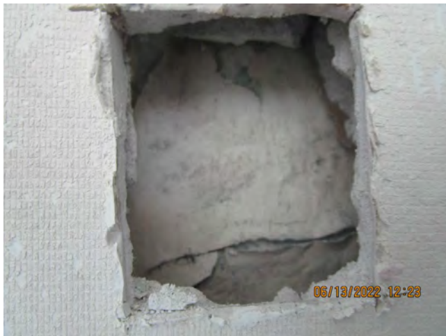
Photographs 8 & 9– 14 th Floor – Plaster Behind Sheetrock and Suspect Mold Growth on Sheetrock Backing Paper
