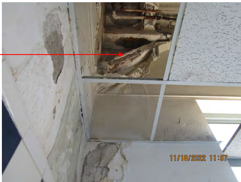
Photograph 3 – 12 th Floor Men’s Restroom Damaged Wall and Ceiling Plaster. Exposed Crossmember Depicted
