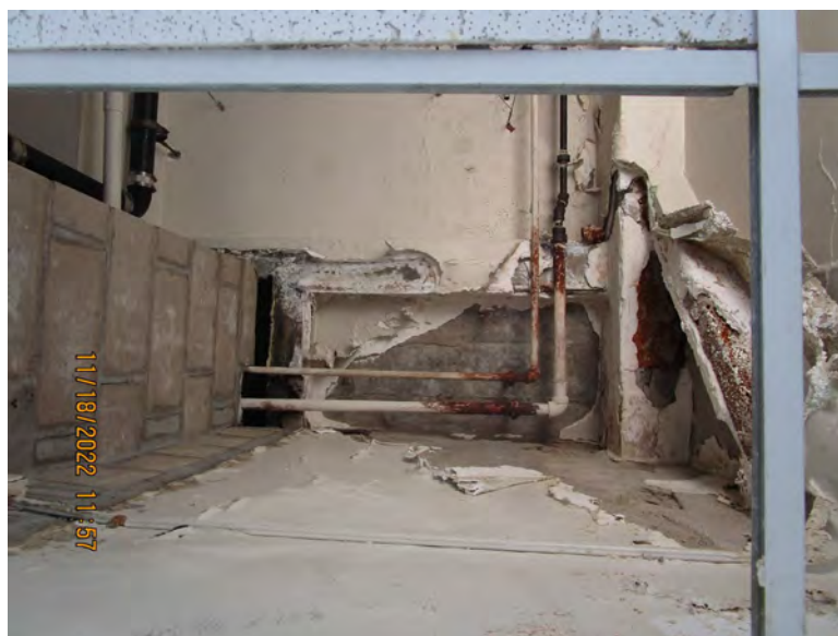
Photographs 4 – 12 th Floor Men’s Restroom Damaged Plaster Ceiling
