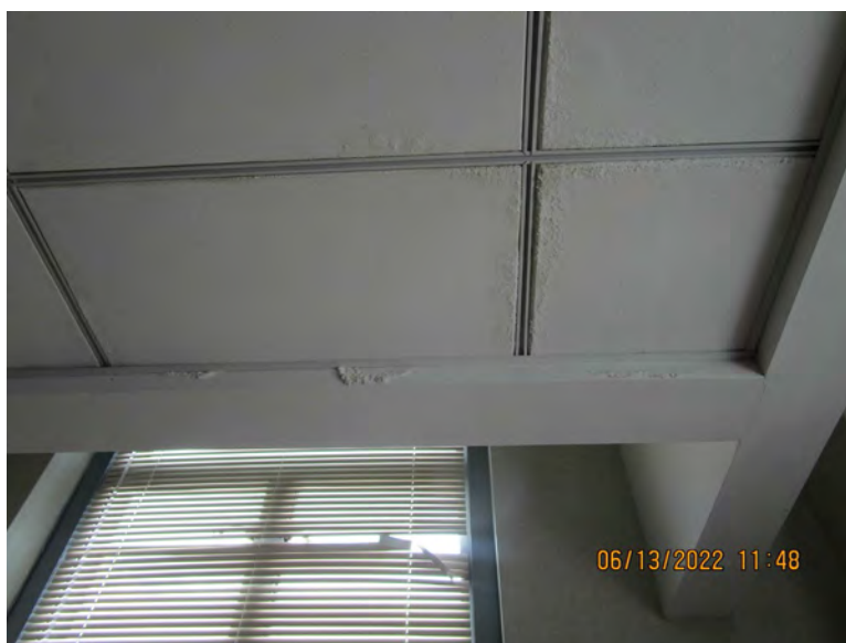
Photograph 6 – 14 th Floor Water Damaged Sheetrock and Ceiling Tiles
