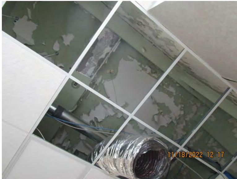
Photograph 10 – 12 th Floor Corner Office Delaminating Paint on Ceiling
