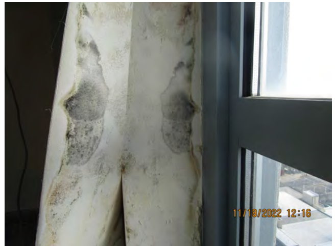
Photographs 6 & 7 – 12 th Floor Corner Office Mold on Wallpaper adjacent to Window
