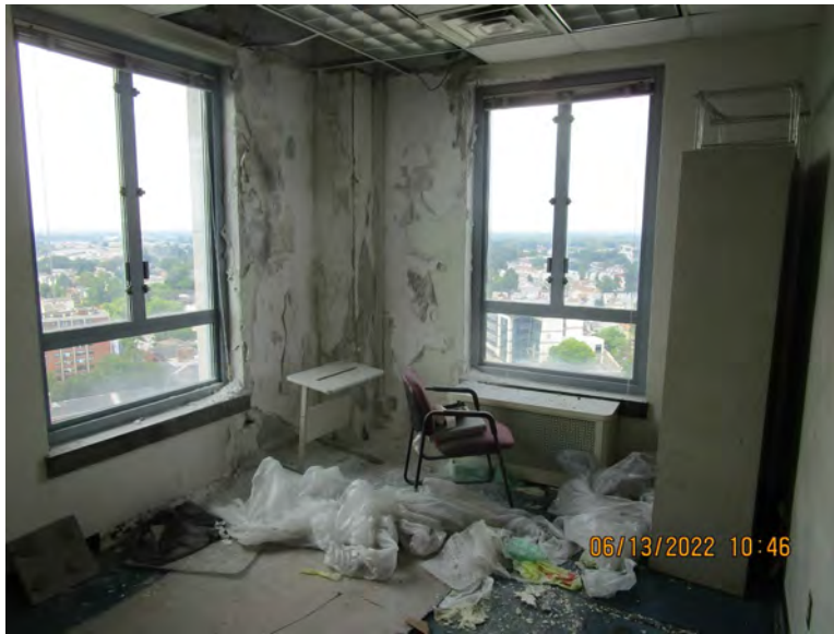
Photograph 1 – 15 th Floor Office Debris and Damaged Plaster
