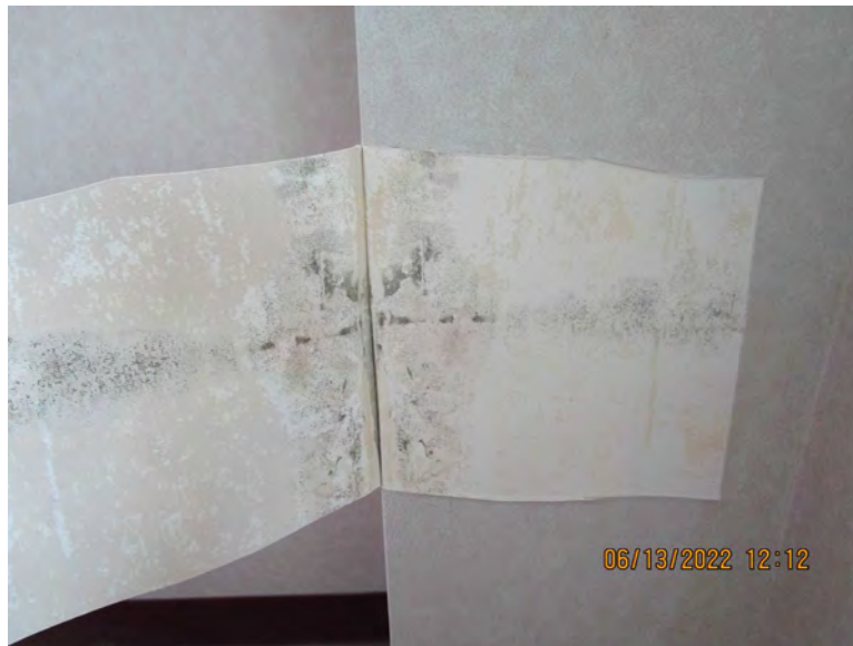
Photograph 7 – 14 th Floor Mold Growth On Sheetrock Behind Wallpaper
