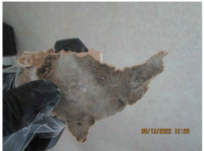
Photographs 8 & 9– 14 th Floor – Plaster Behind Sheetrock and Suspect Mold Growth on Sheetrock Backing Paper
