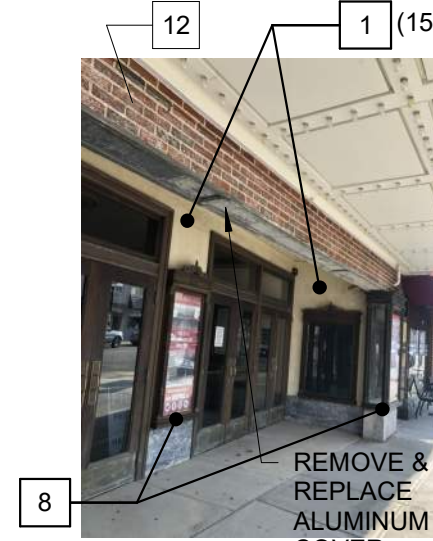
12 1 (150 SF.) 8 REMOVE & REPLACE ALUMINUM COVER 10 PHOTO DETAIL 10
