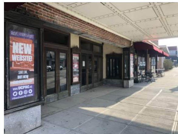
1 PHOTO DETAIL 01 OVERALL VIEW OF EXTERIOR
