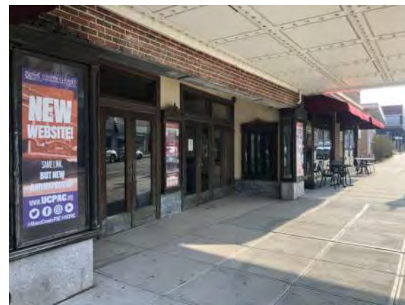
1 PHOTO DETAIL 01 OVERALL VIEW OF EXTERIOR
