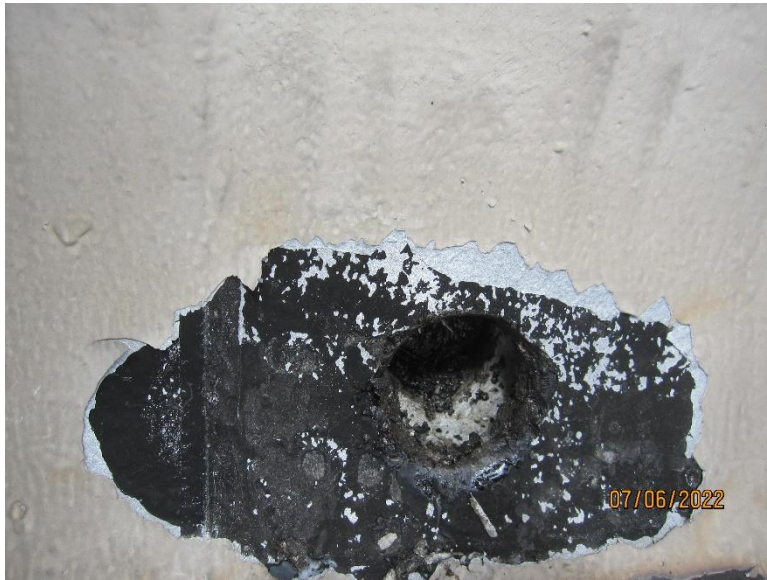
Photo 11 - Probe RP3 - View of the removed probe sample.
