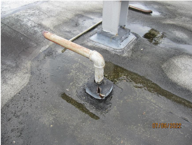
Photo 6- View of open operational pitch pocket located on the penthouse roof.
