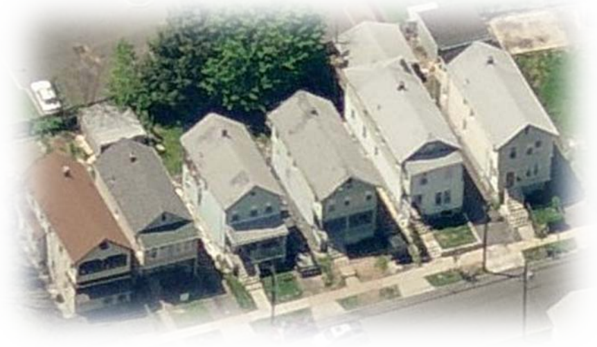
Photo 8-5: Example of Two Family High Density Residential
