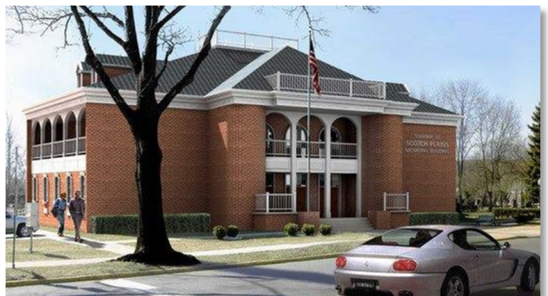
Scotch Plains Municipal Building. Source:
